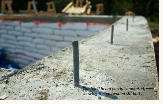
The next day when the concrete had set the forms were unscrewed and popped off, and then positioned over the next section of wall. This procedure was repeated, adjusting the forms for fit, and building up forms for each corner, until a solid bond beam was completed around the entire perimeter.
