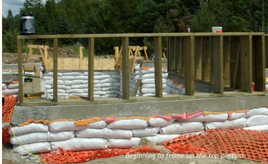
With the sill board in place the framing carpentry began. Everything was overbuilt where possible, to prepare the roof for the heavy load of soil, moisture and snow which would eventually be on top of it. The walls were then sheathed with exterior plywood and painted to seal them from the weather.
